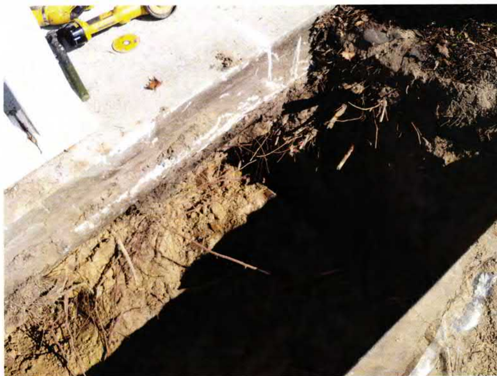
Picture 2: UST 219Balsam excavation.
